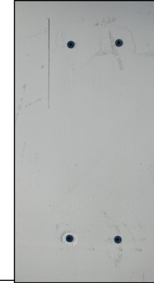
Step 3: Install anchors
